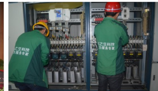
Engineers conduct on-site inspection
